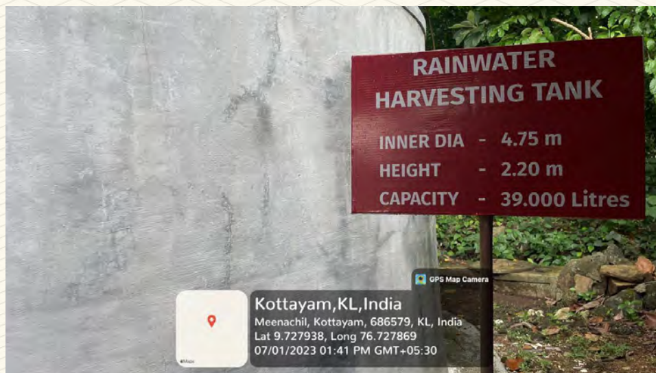
Figure 9: Rain Water harvesting tank Photo 2
