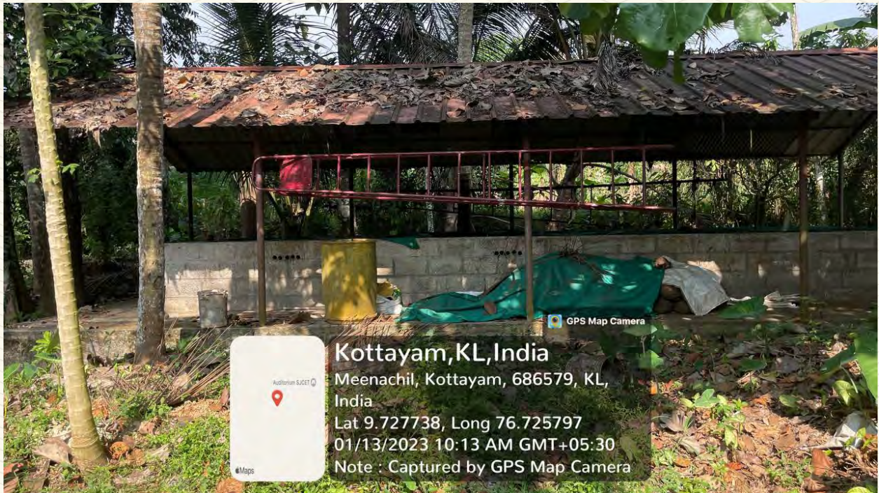
Figure 75: Waste management plant photo 2
