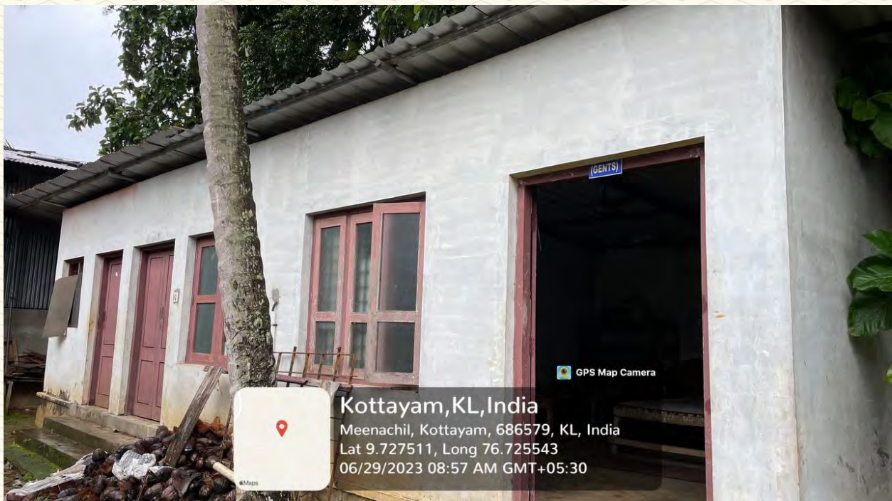
Figure 127: Labours Rest Room Photo 1
