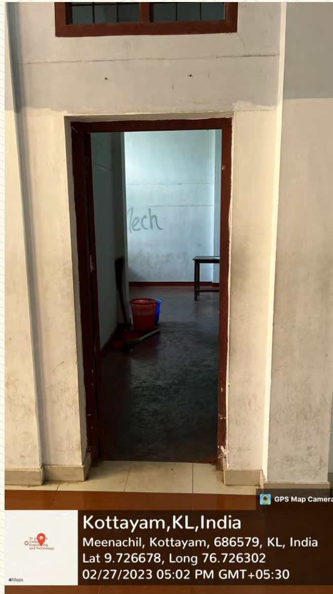
Figure 170: Gents waiting room Photo 1
