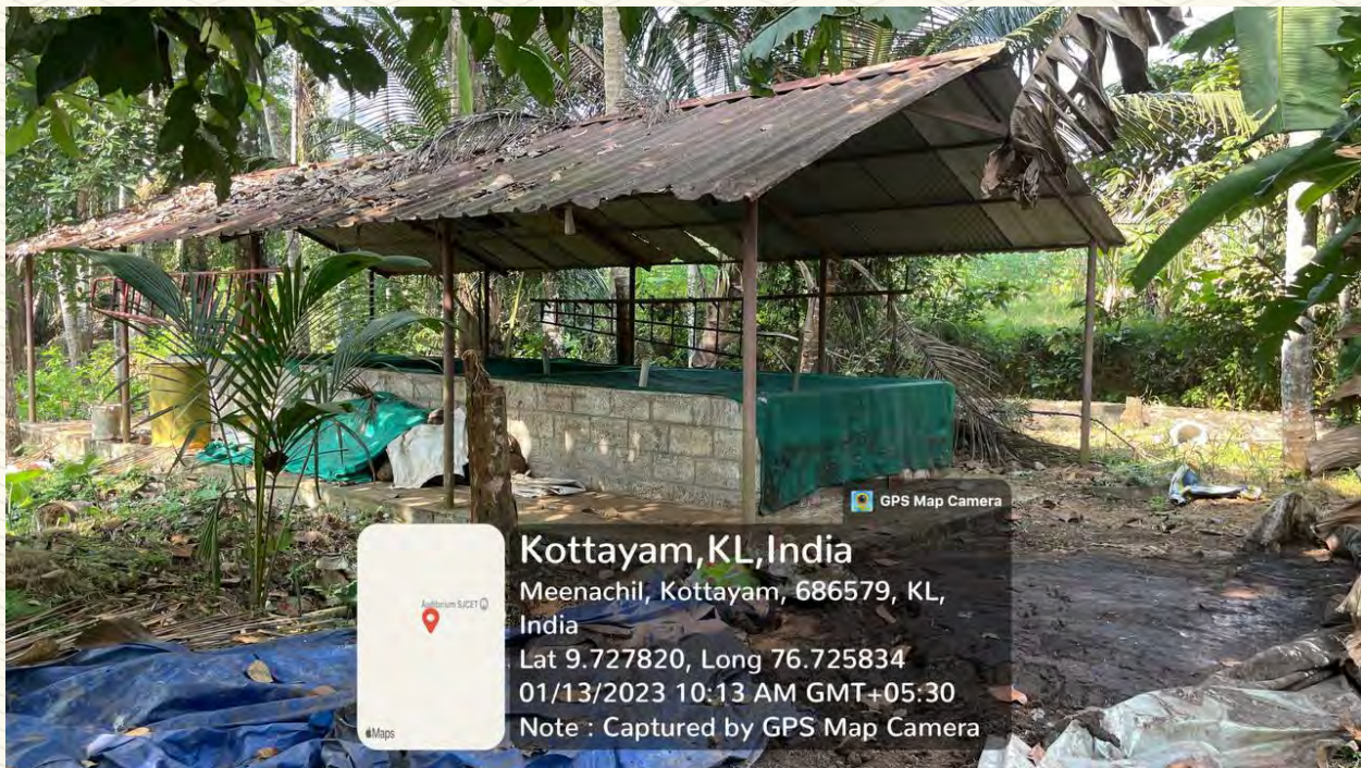
Figure 74: Waste management plant photo 1
