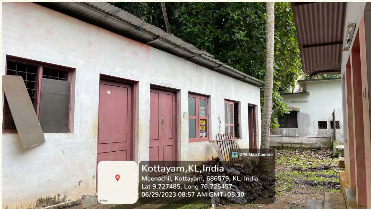
Figure 129: Labours Rest Room Photo 3
