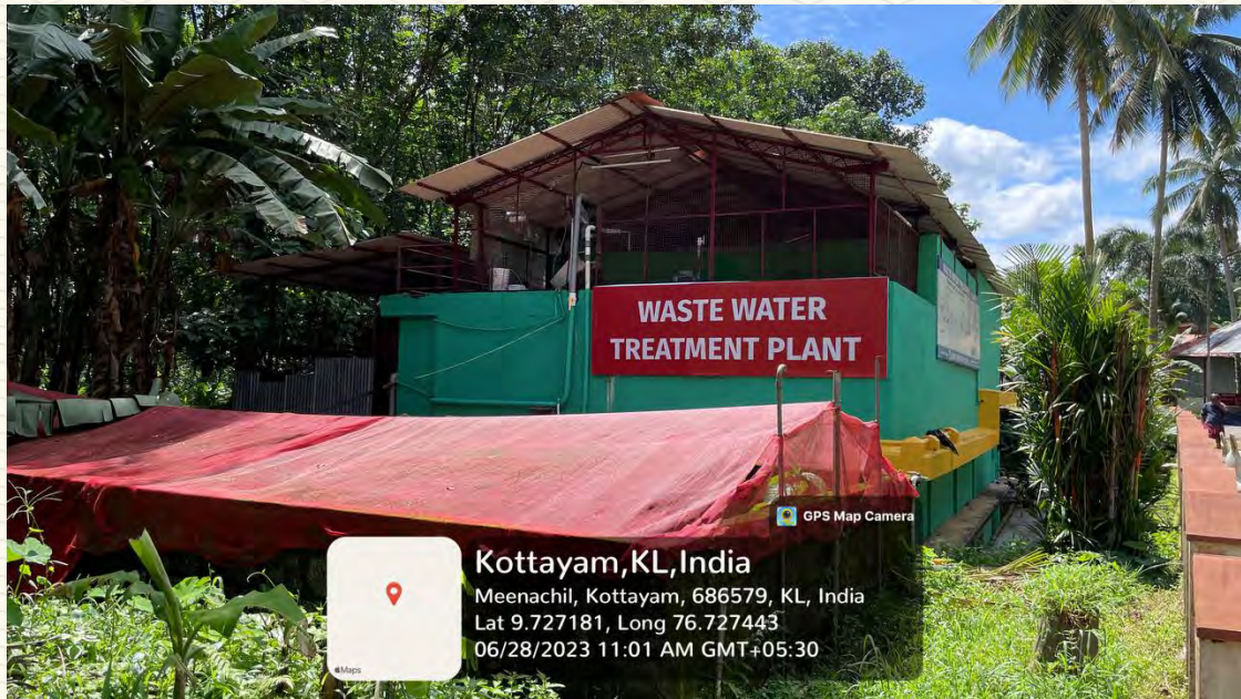
Figure 77: Waste water treatment plant Photo 1
