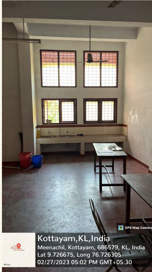
Figure 172: Gents waiting room Photo 3
