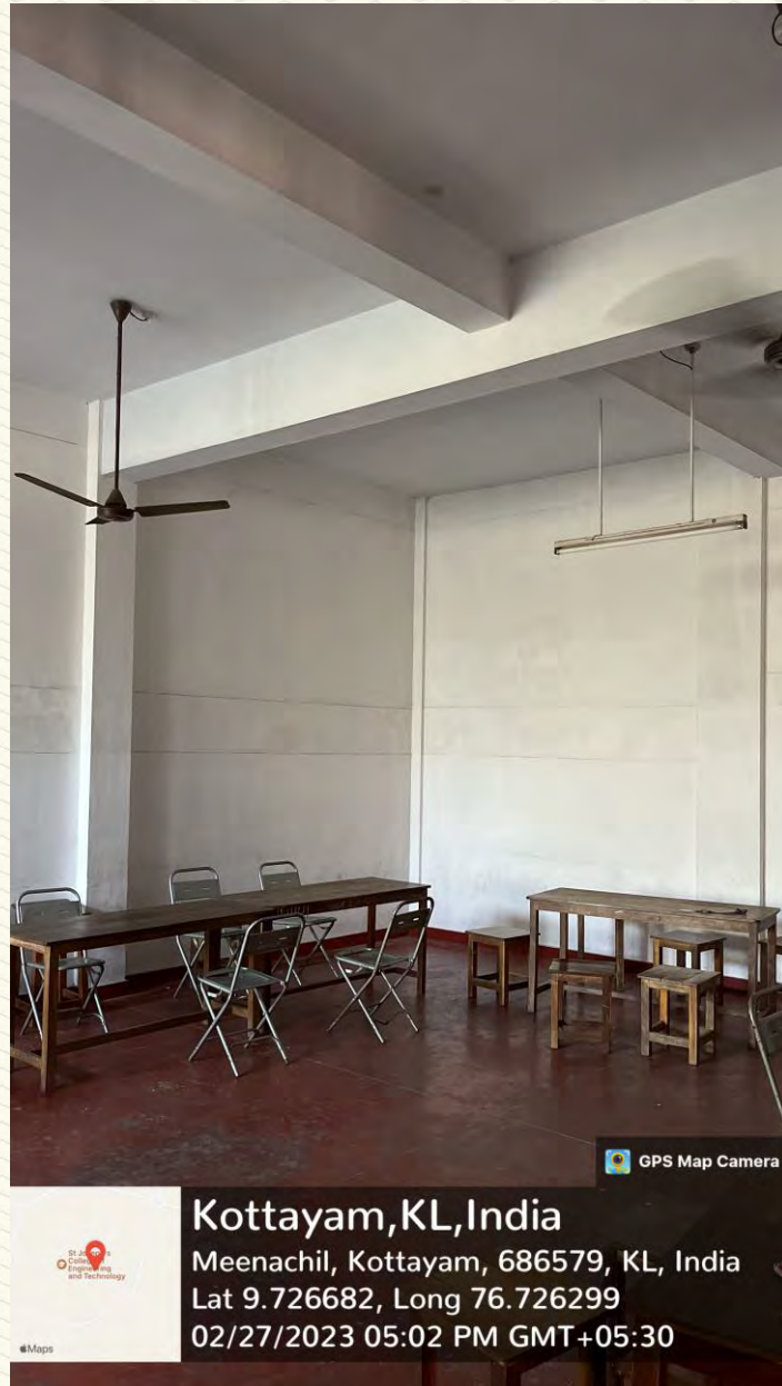
Figure 171: Gents waiting room Photo 2
