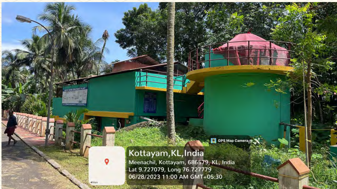
Figure 78: Waste water treatment plant Photo 2
