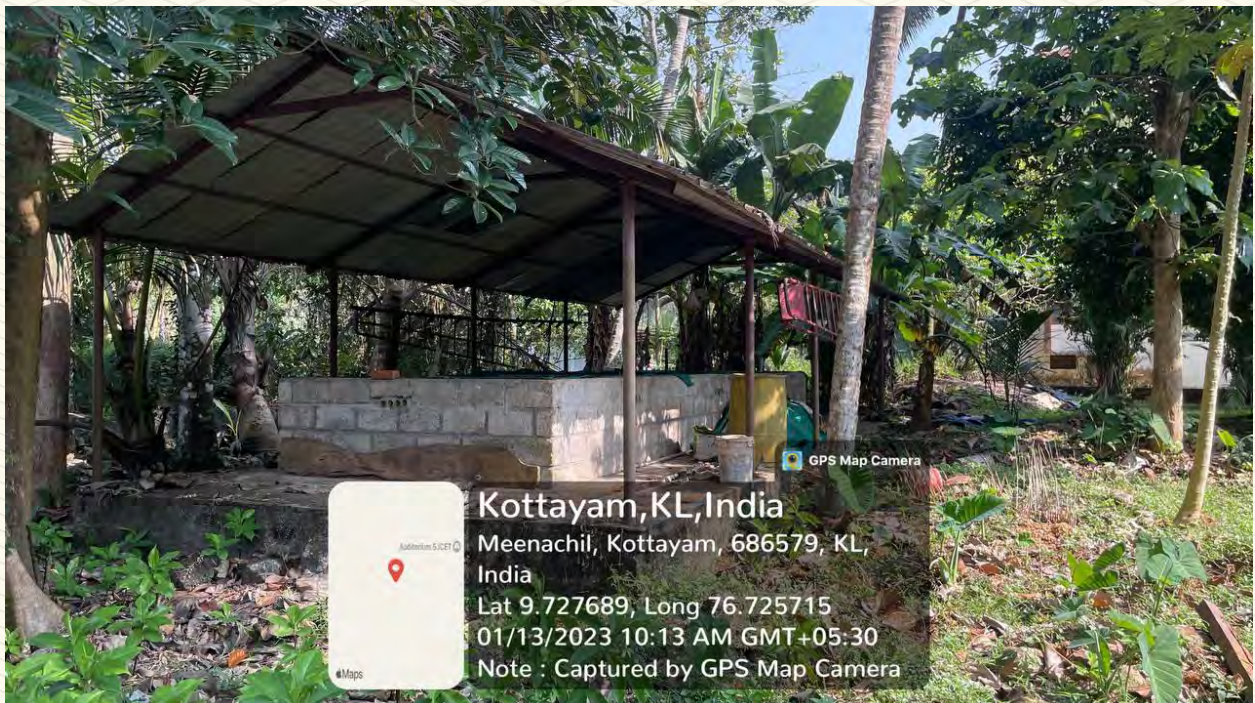
Figure 76: Waste management plant photo 3
