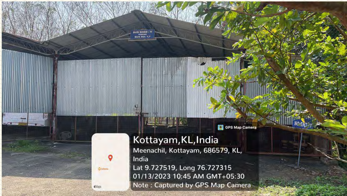
Figure 142: Bus Shed photo 5
