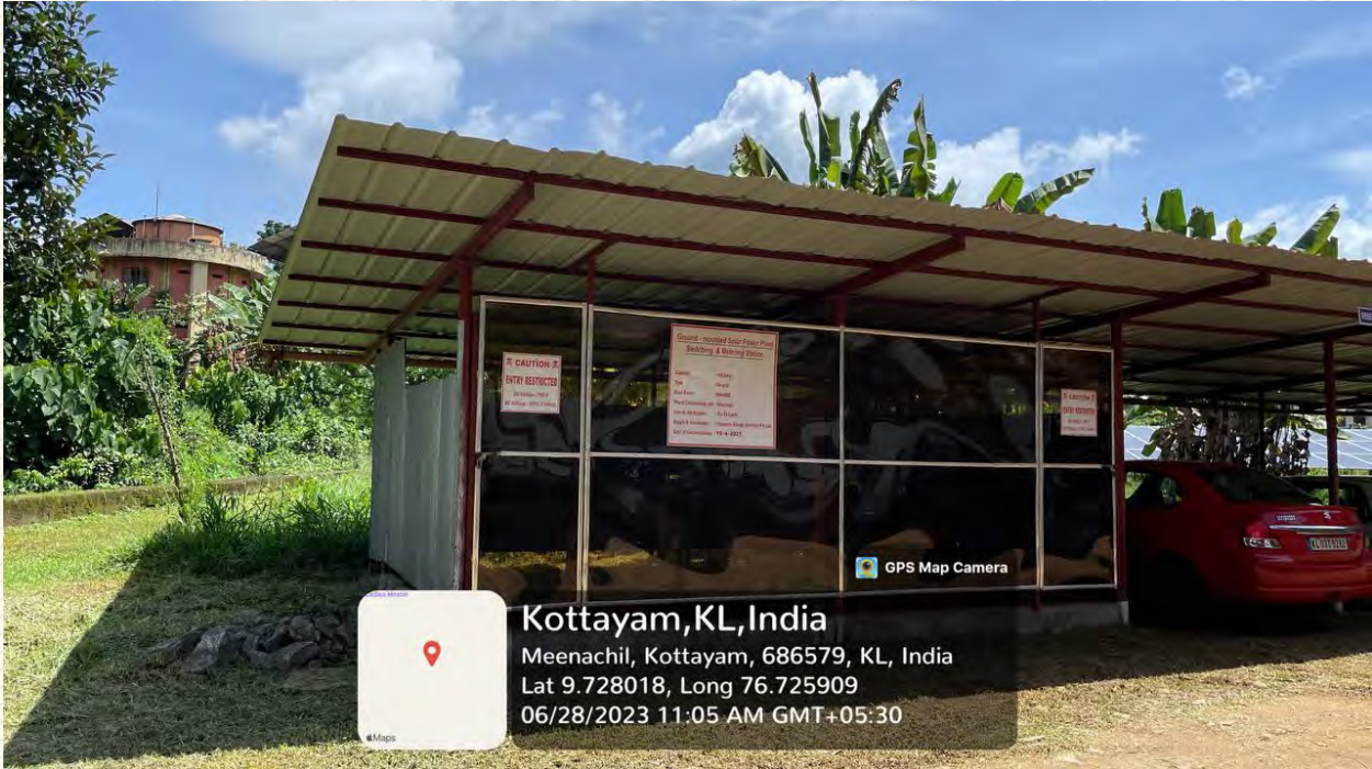
Figure 97: Ground -Mounted Solar Power Plant Photo 2
