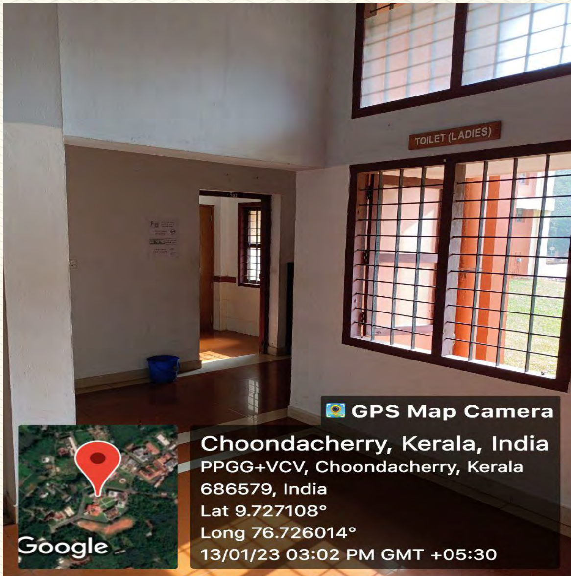
Figure 13: Ladies Toilet Photo 1
