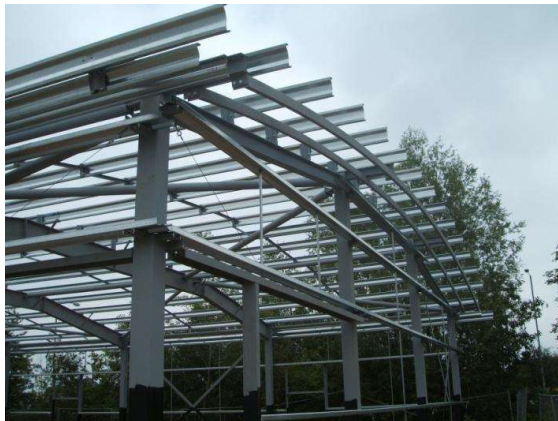
Fig -1: Cold Formed Steel Structures
