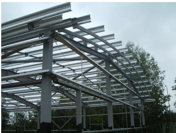
Fig -1: Cold Formed Steel Structures
